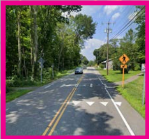
Church Street (Rte. 85)
