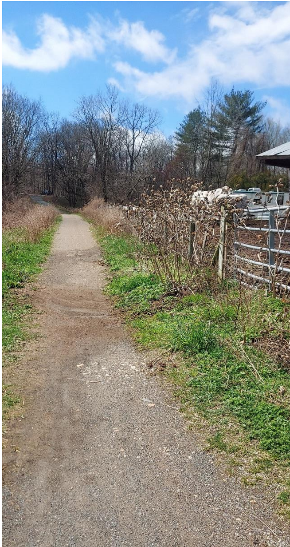
Figure 12 Manure contaminated stormwater flows across the Airline Trail from an adjacent farm.
